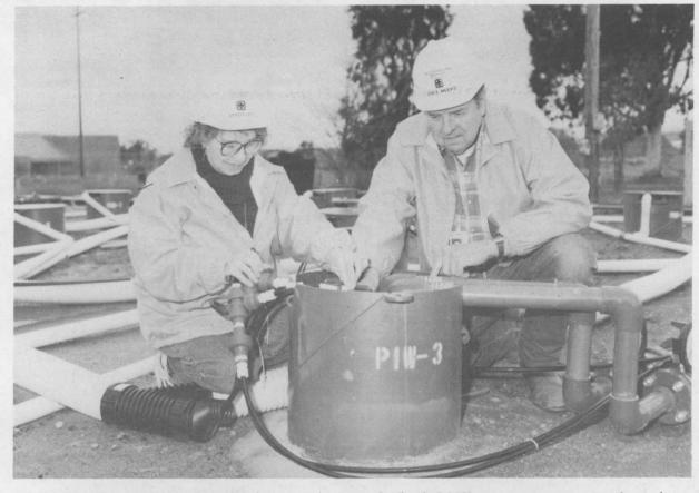
BIOREMEDIATION WELLHEAD — Sandy Leo and Jon Meeks (both 8642) prepare to pump nutrients down one of four wellheads used for aeration and nutrient injection at the fuel oil spill site being cleaned up through a bioremediation technique.
